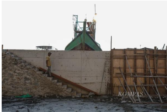
Figure 2. The Construction of a 3.6-Meter Coastal Embankment in Pluit. Source: (Fadlurrohman, 2025)
