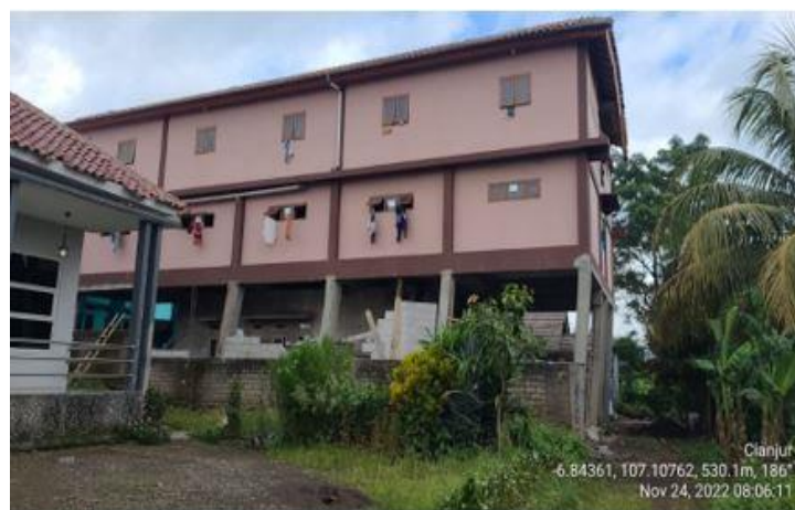
Figure 3. (Left) Minimarket building & (Right) 2-3 storey building
